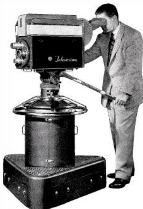
CAMERA is counterbalanced in Model PD-3 TV Pedestal by Houston-Fearless, enabling cameraman to raise or lower with ease.
